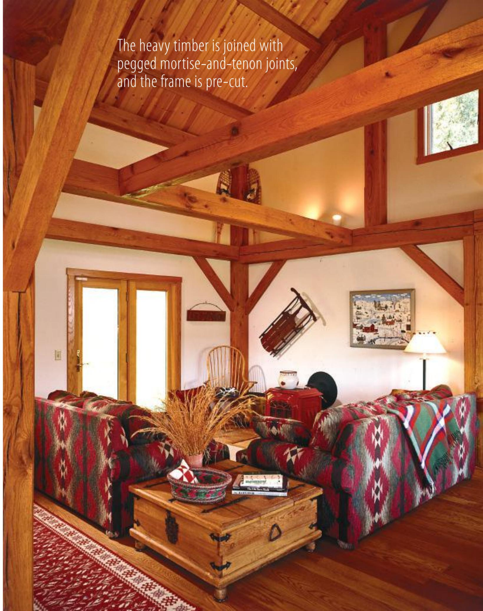
The heavy timber is joined with pegged mortise-and-tenon joints, and the frame is pre-cut.
