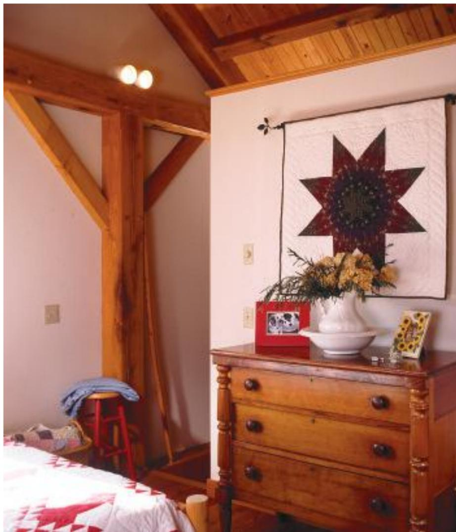
using hand-held power tools instead of the usual computer numerical-control machinery. "This allows us to do tighter joinery," Johnny explains. "Our focus is on exceptional craftsmanship, and we are known for paying attention to detail. Our joints are pinned with hickory dowels with offset holes so when the pin is driven, everything is pulled extremely tight. And we have incredible quality control because the same crew that crafts it installs it. And everyone who works on it is in our family."
