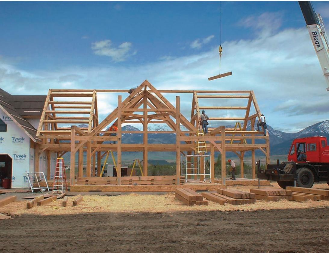
The timber frame nears completion. Tradition dictates that the homeowners—and crew members—sign and date a peg or two before they're driven in. When the frame is fully finished, a small evergreen tree is nailed to the frame's peak to celebrate and honor the trees that live on in the timbers. Although a frame standing alone is a thing of beauty that begs to be admired, it must be enclosed in order to create a livable home.
